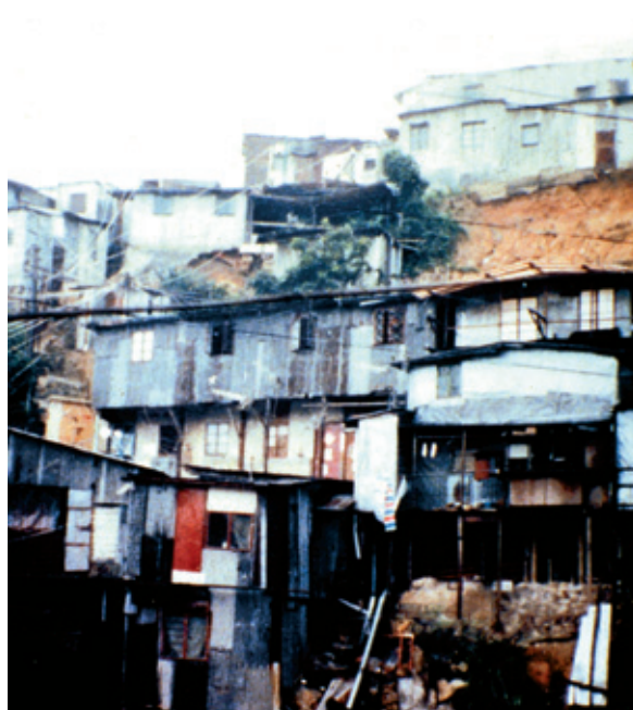
Urban development on steep land in Hong Kong. Aerial view of the same site after a landslide triggered by heavy rains.
